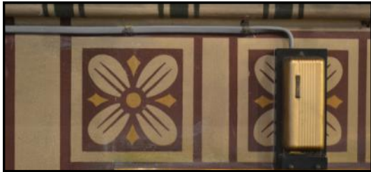
Defunct thermostat/wiring removed and damage repaired
