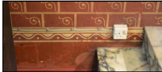
Electrical socket to be more discreetly located and damage repaired
